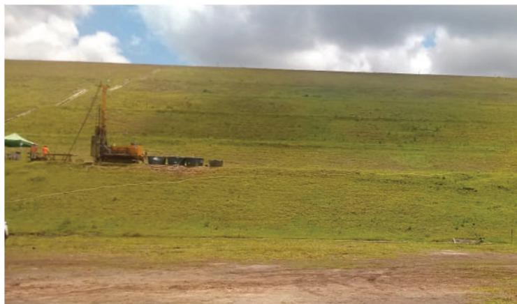
Fig. 3. Vale's drill-rig operating on the sloping berm of Brumadinho Dam drilling through the embankment and tailings (photo by Mr A Fanaya one week before failure).
