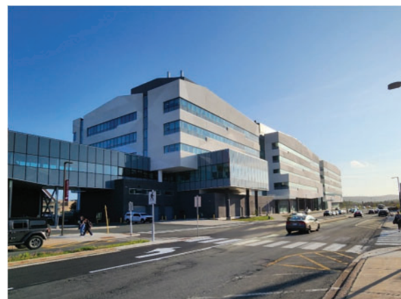
Fig. 1. Core science facility building.
